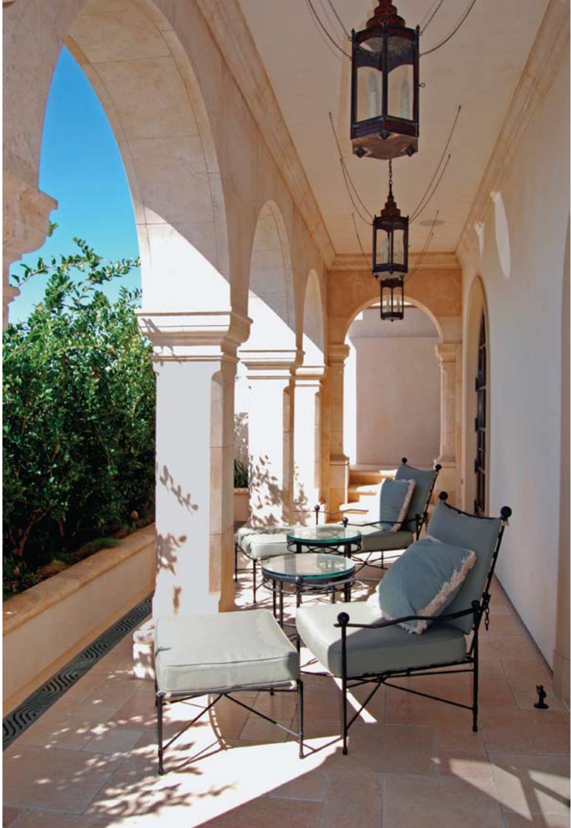
Massangis limestone was also used for columns, wall claddings and cornice and corbels, as well as for balcony flooring.
